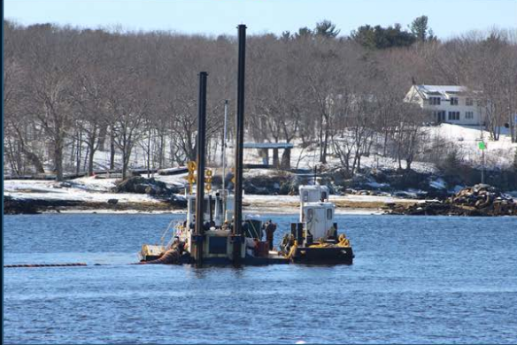
Saco River Dredging
